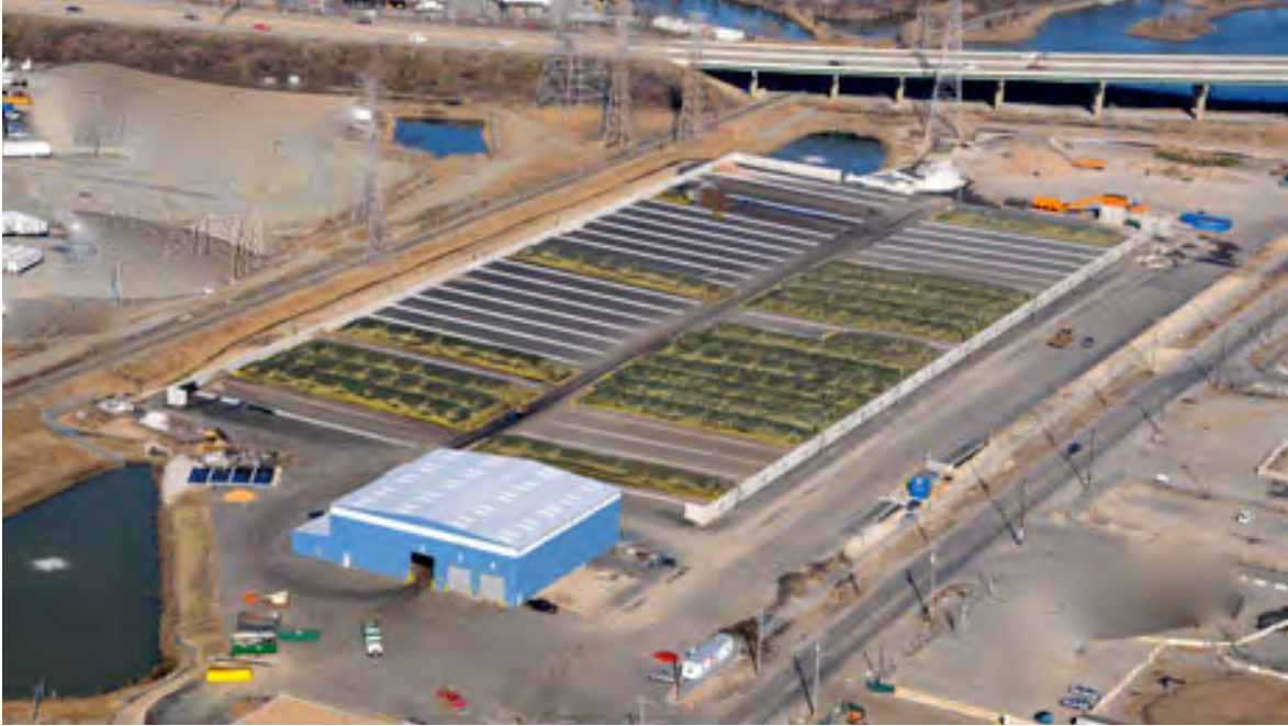
The Wilmington, DE, Organic Recycling Center, run by the Peninsula Compost Group. Opened in 2009, it can compost 160,000 tons of material annually. http://peninsula-compost.com/facilities/WORC.html
