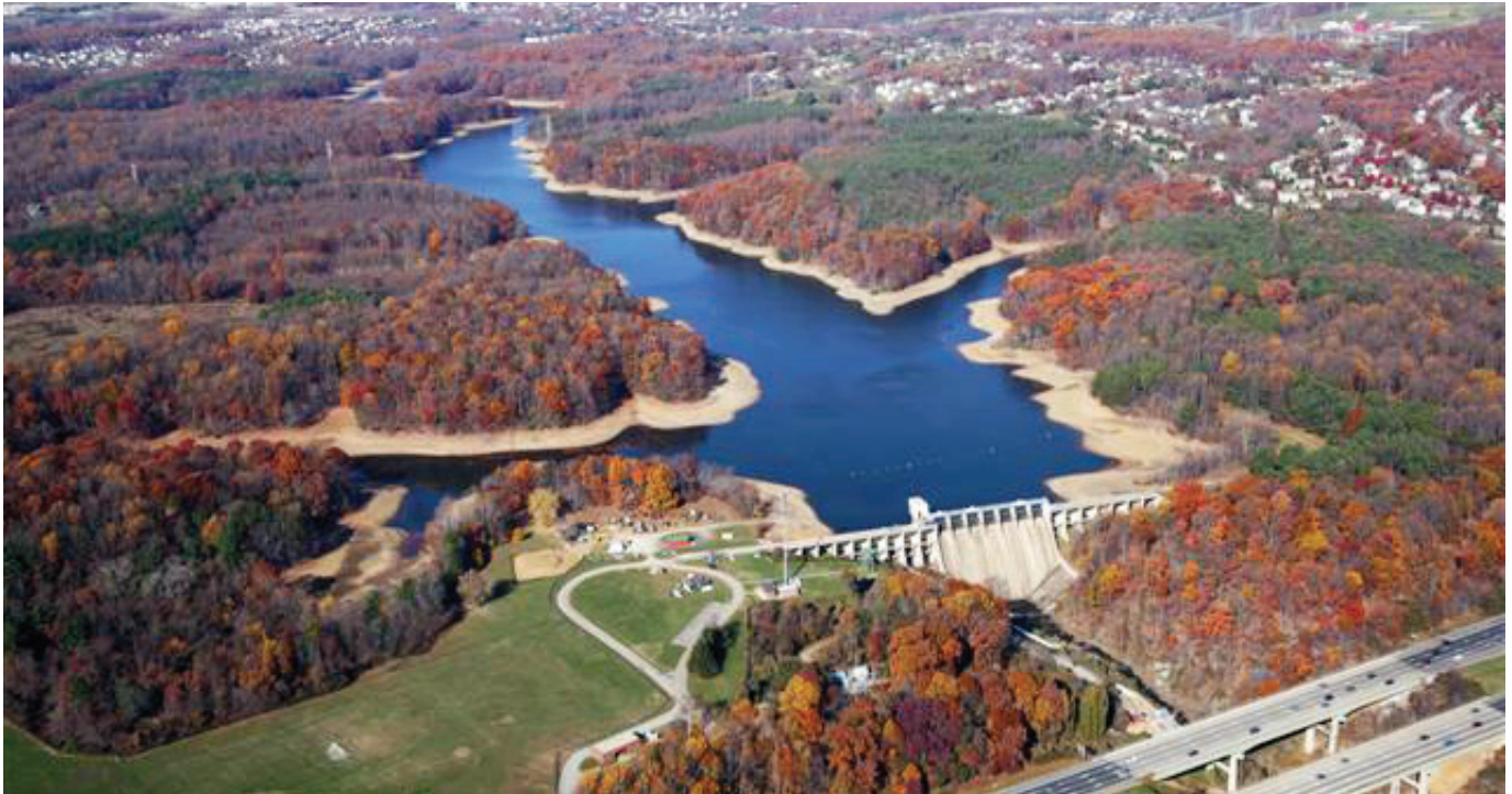
Washington Suburban Sanitary Commission's T. Howard Duckett Dam on Rocky Gorge Reservoir, Howard and Prince George's Counties
