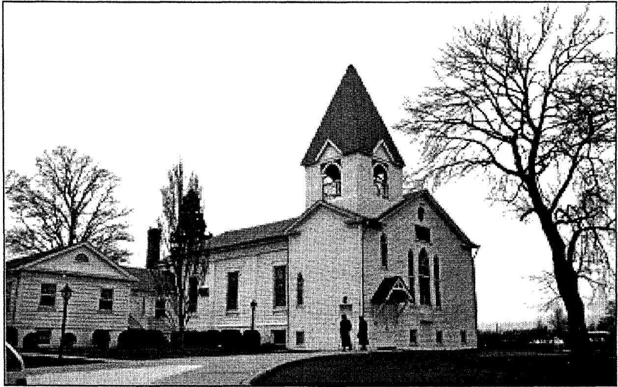
24/19-1 Darnestown Presbyterian Church (1856, 1897) 15120 Turkey Foot Road
