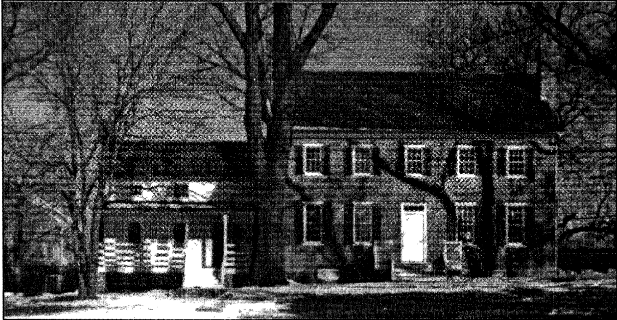
29/16 Locust Grove I (c1773) 7340 Westlake Terrace
