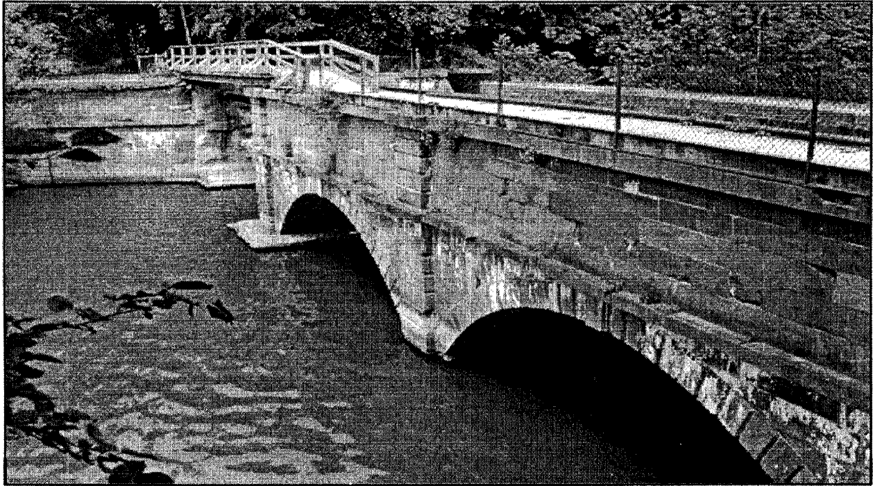
24/25 Seneca Aqueduct (1831) Mouth of Seneca Creek
