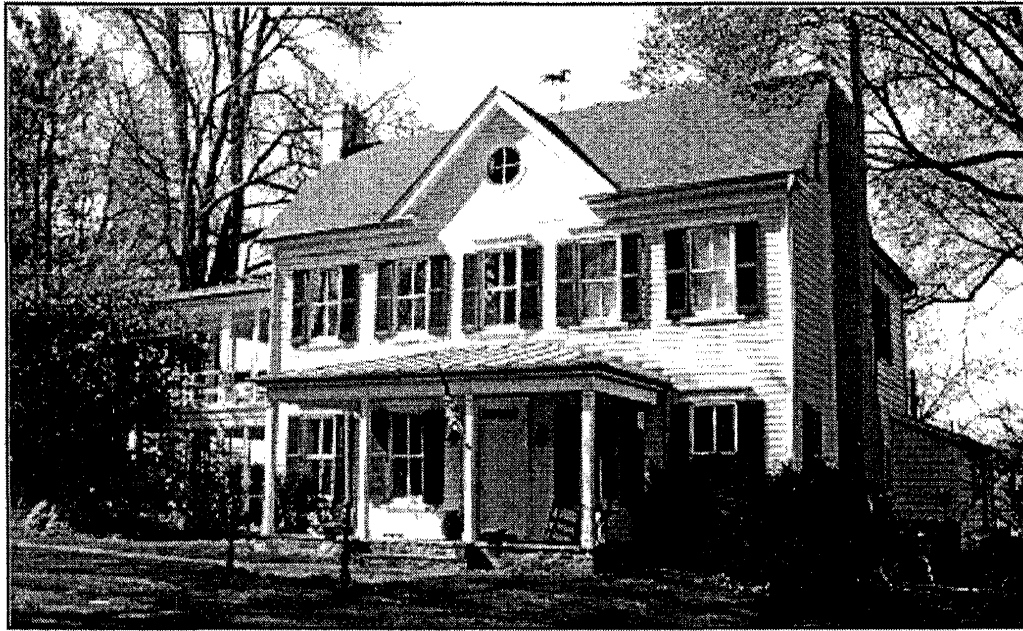
29/7 Capt. John McDonald House (c1873) 10600 River Road
