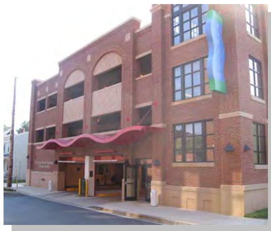
Knighton Parking Garage
