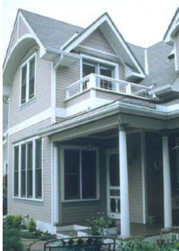
Plan BC-1700 reminds passersby of the simple homes their grandparents owned. Inside, an updated floor plan responds to modern lifestyles.
