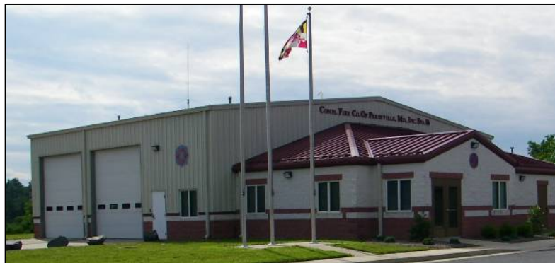
Perryville Fire Company building on MD 222 near I-95
