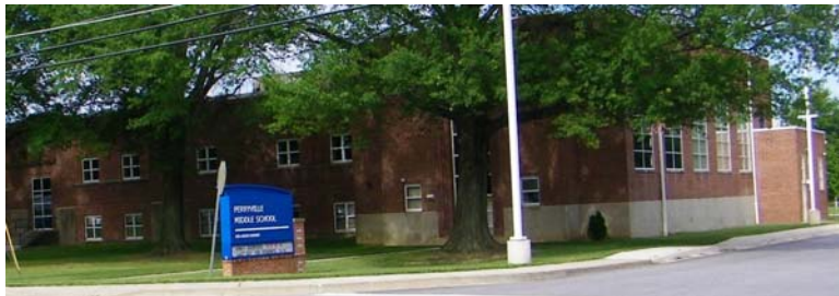
Perryville Middle School. In Cecil County adequate public facilities requirements will be most applicable to schools.
