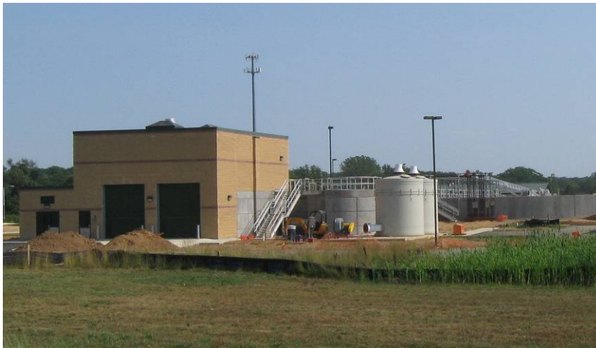
Elkton Wastewater Treatment Plant is owned and operated by the Town of Elkton.
