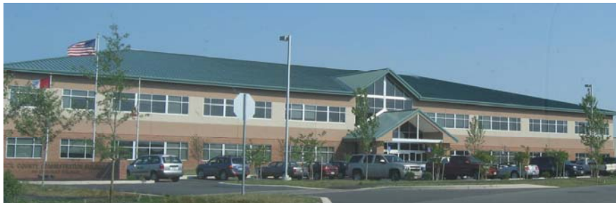
The new 83,000 square foot County Administration Building opened in 2008
