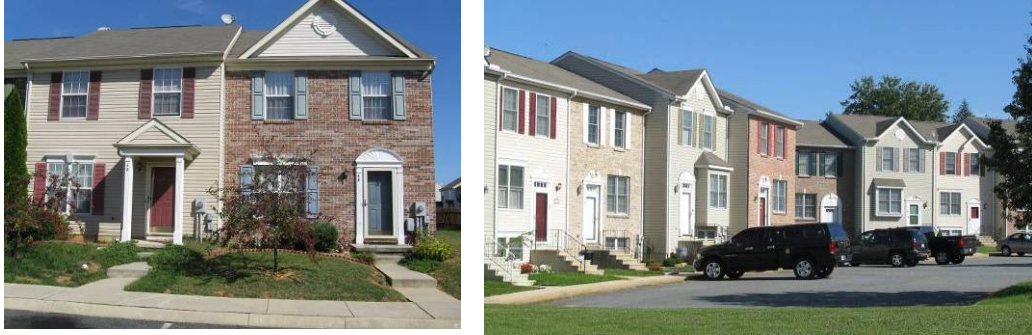
Housing is considered high density at 8.34 units per acre in Whitehall West subdivision (right) and at 11.23 units per acre in Chesapeake Landing (left).
