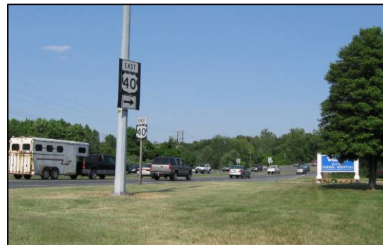
U.S. Route 40 Eastbound at MD 279
