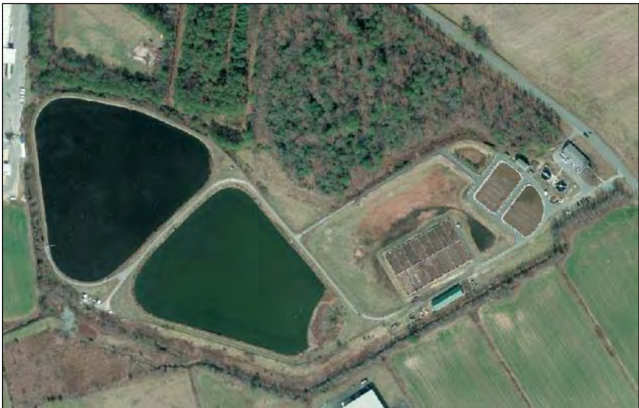
Photo 5-2: Denton Wastewater Treatment Plan, 650 Legion Road, Denton, MD
