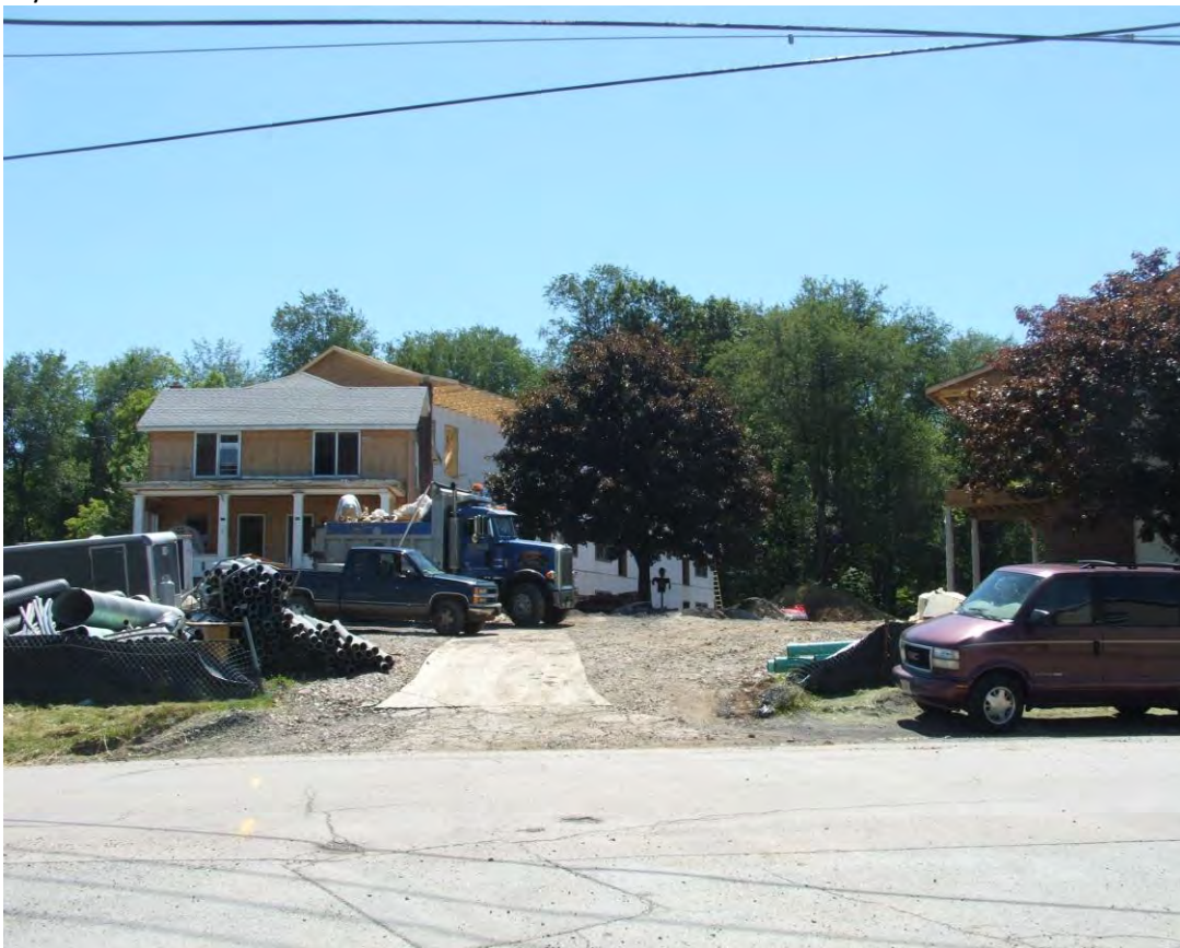
Welsh Hill Commons, Infill Student Housing Under Construction 2008
