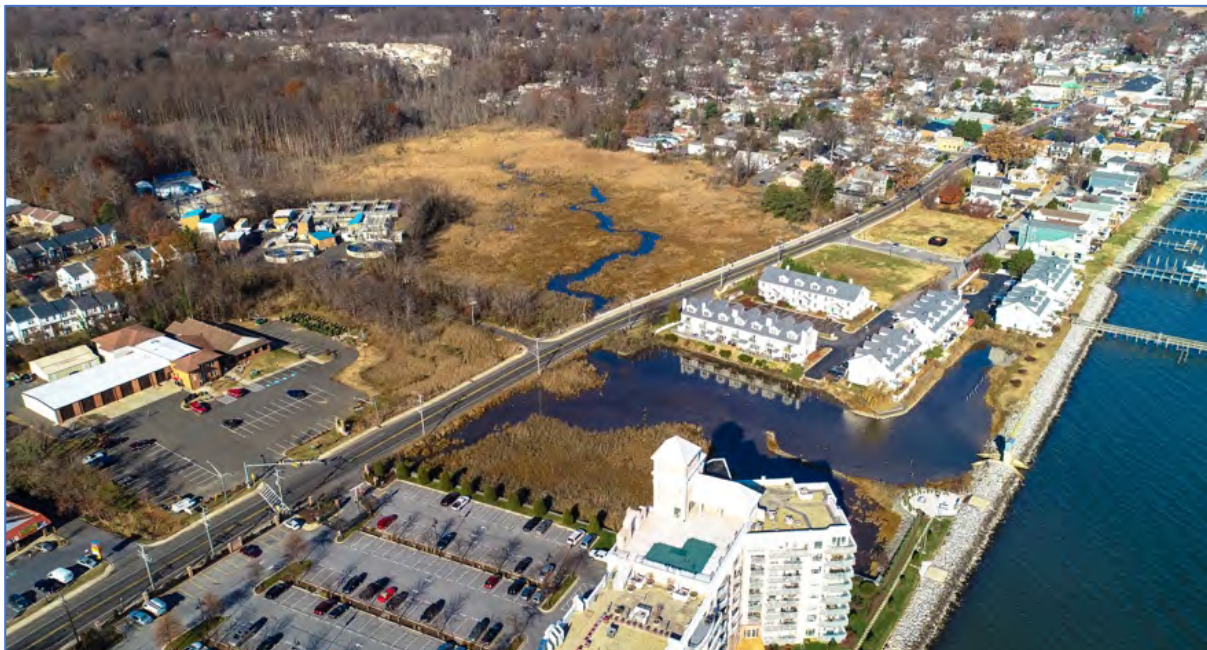
The 12.5 acre Estuarine and Marine Wetland on the west side of Bayside Road and the growing open water west of the sea gate.
