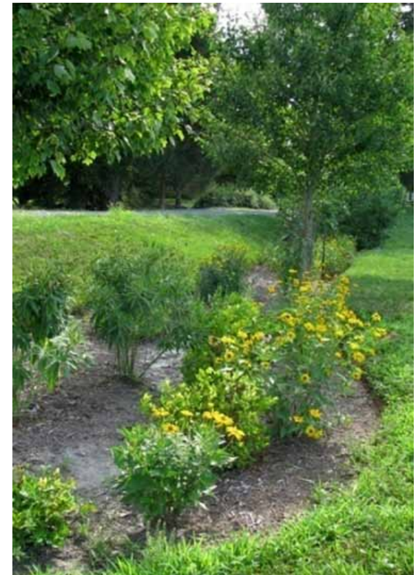
Environmental Site Design techniques, such as this rain garden, are required by the new stormwater management regulations.
