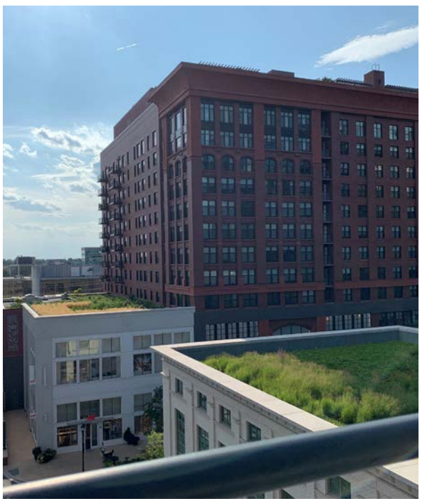
A green roof.
