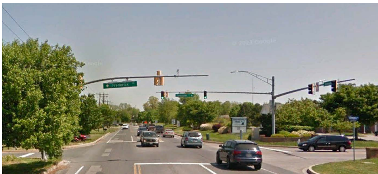
FIGURE 12: MD ROUTE 213 AT THE COURSEVALL INTERSECTION
