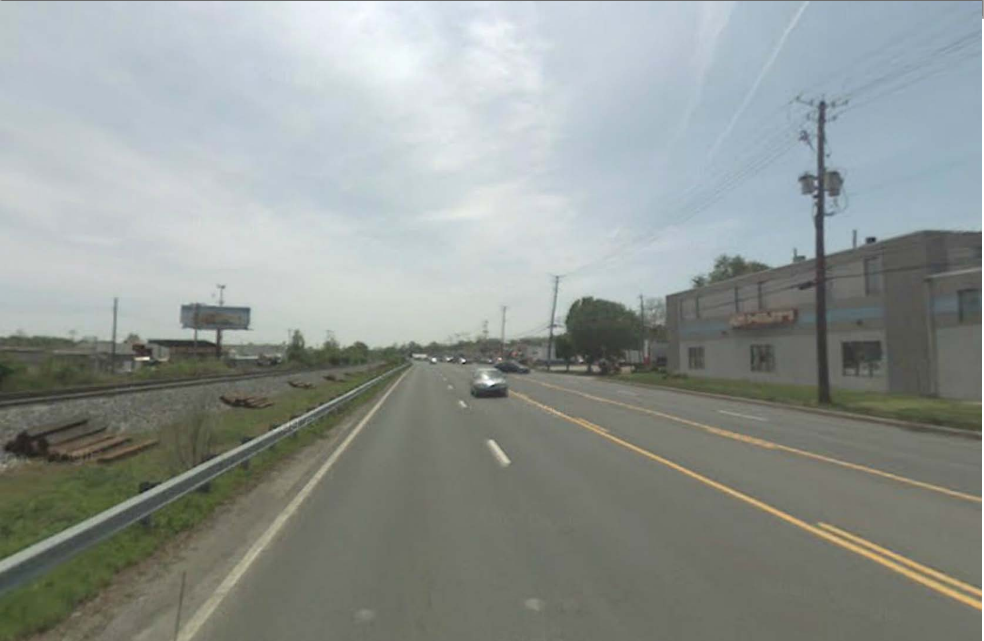
Route 1 south of Laurel building/road/ rail
