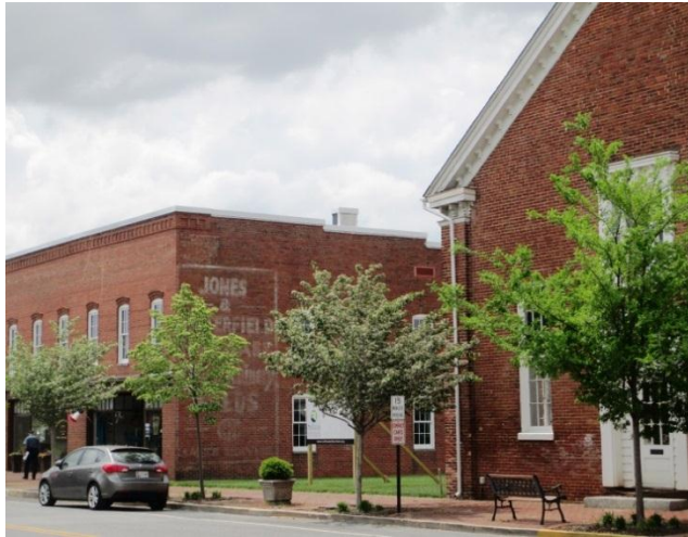
Site of the future Platinum LEED Sultana Education Foundation Education Center
