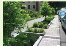
▲ EXAMPLE: A residential "curbless" street example that allows stormwater runoff to sheet flow into a continuous green gutter system. The sidewalk is also constructed with pervious concrete.
