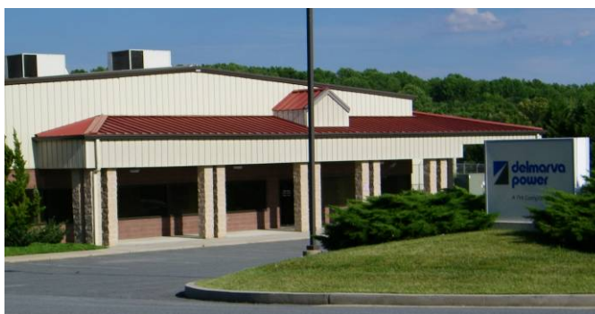
North East Commerce Center offices of Delmarva Power, which provides power for much of Cecil County.
