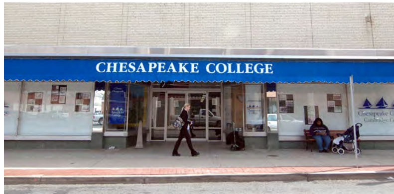
MEDCO purchased a former two-story Cambridge department in from the Dorchester County Commissioners using a $1 million loan from the Maryland Industrial and Commercial Redevelopment Fund program of DBED. MEDCO leases it to Chesapeake College as an adult education and industrial training center. MEDCO's purchase completed more than two years of state and local development efforts to convert a large empty structure in the downtown and stimulate job creation.
