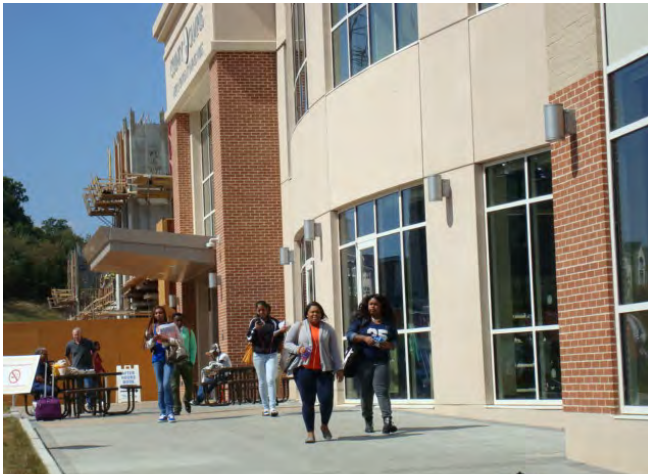
Metro Centre at Owings Mills transit oriented development, a public-private partnership, partially funded by TIF, contains the county’s largest library branch. The Community College of Baltimore County shares the six-story, 120,000 square foot building, built to meet LEED Silver green building standards.
